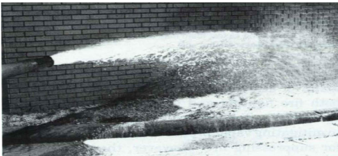
Figure 7.19 The foam nozzle mixes air with the foam concentrate to produce an effective foam blanket.
